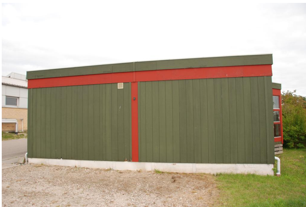
Figure B.3: The west facade.
