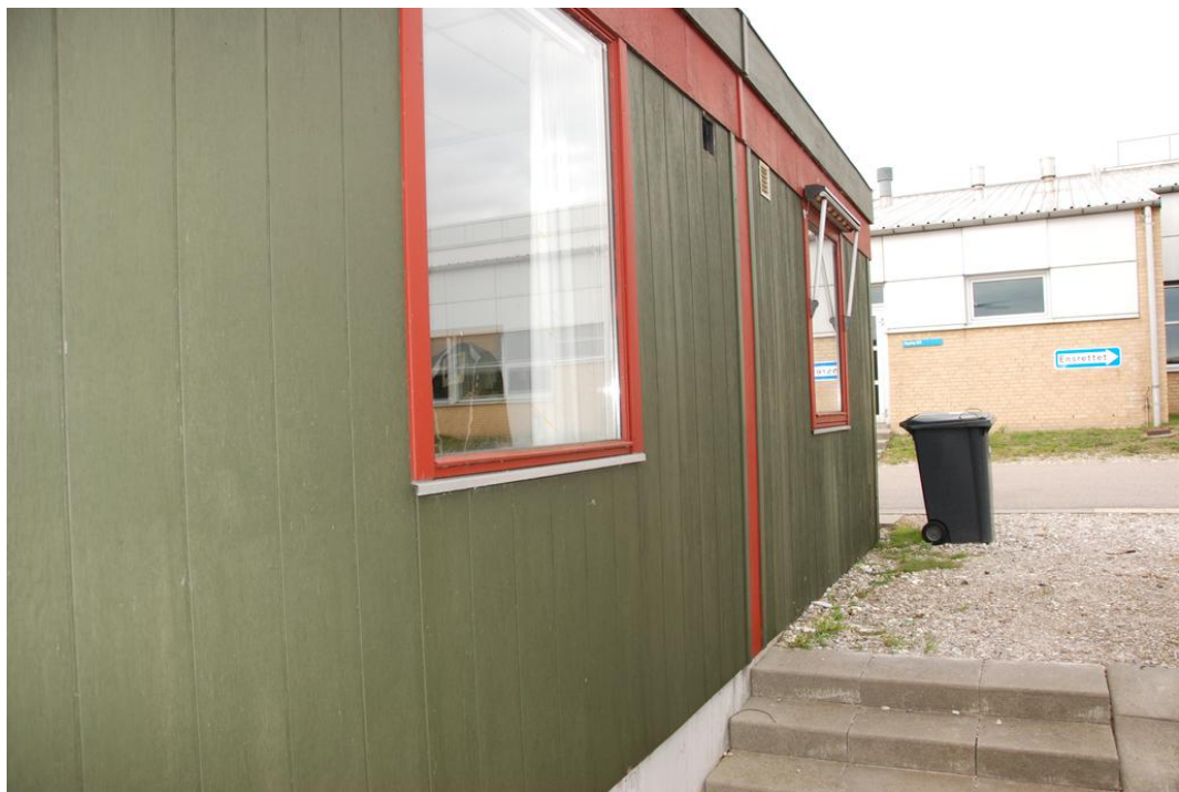
Figure B.1: The east facade.
