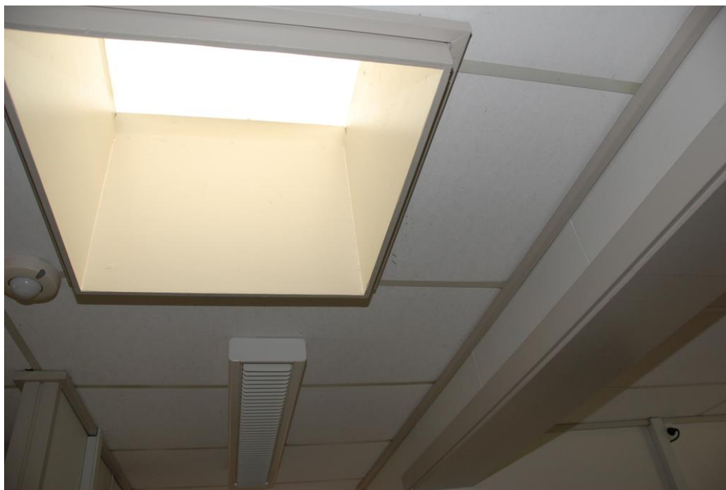
Figure B.9: Window in the ceiling.
