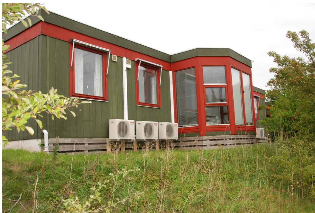
Figure B.2: The south facade.
